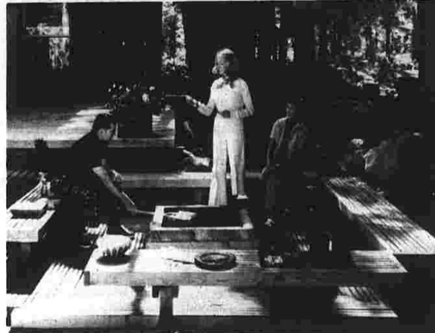
An expansive deck with sunken firepit and surrounding benches makes this backyard addition a center for family entertaining. The deck and benches were built using 2x4s of western wood framing lumber. The firepit is made of concrete blocks. A wood cover converts the firepit to a table top.
