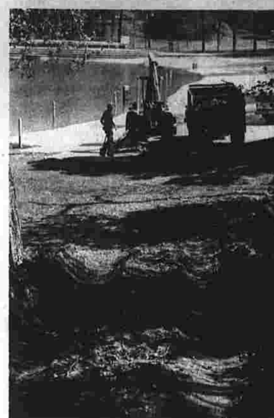
Globe Hollow project under way
